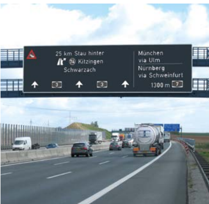
Modern motorway guidance system
