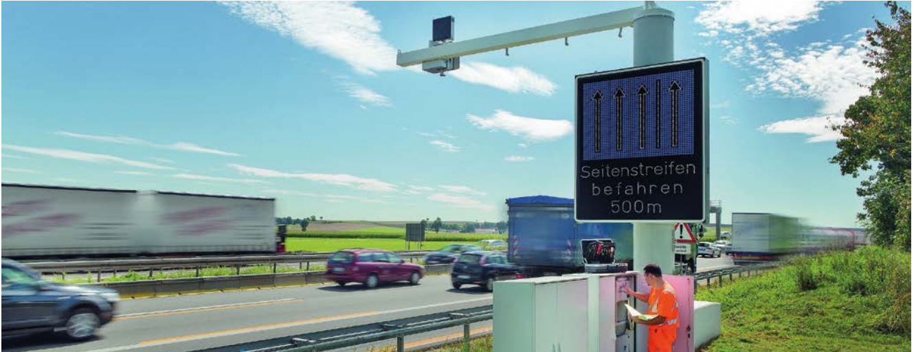
The flexible use of the hard shoulder increases motorway capacities at peak hours
