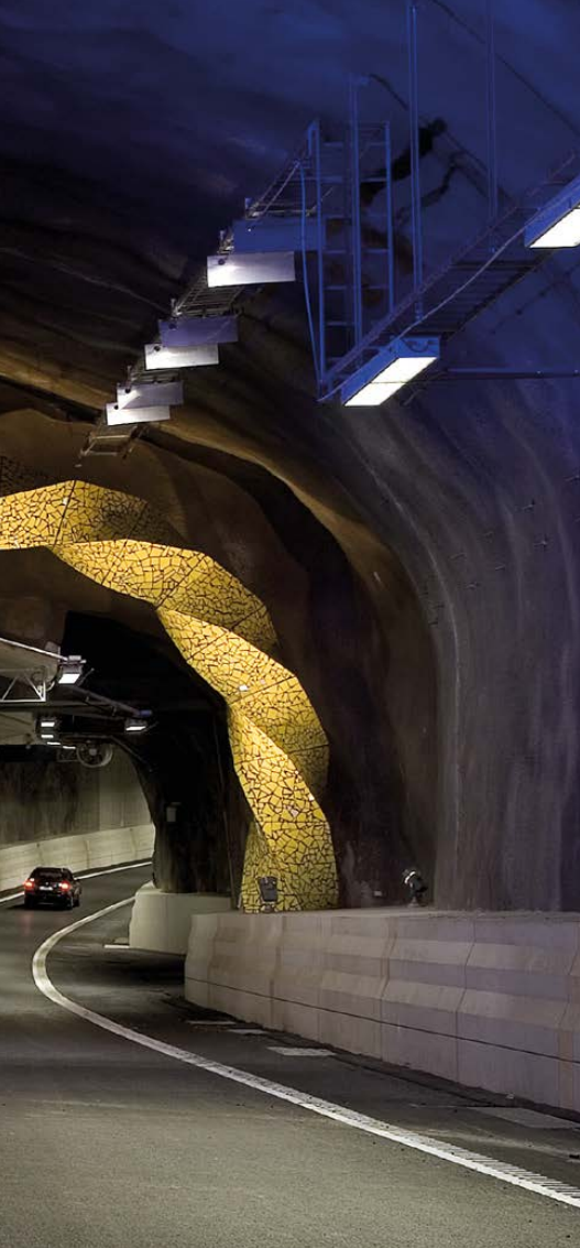
A look into Stockholm's underground motorway link Södra Länken
