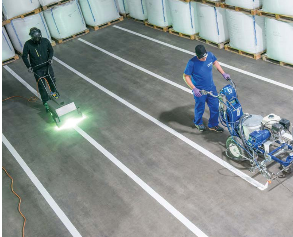
SWARCO UV-LINE: A novel ultra-fast curing indoor marking system
