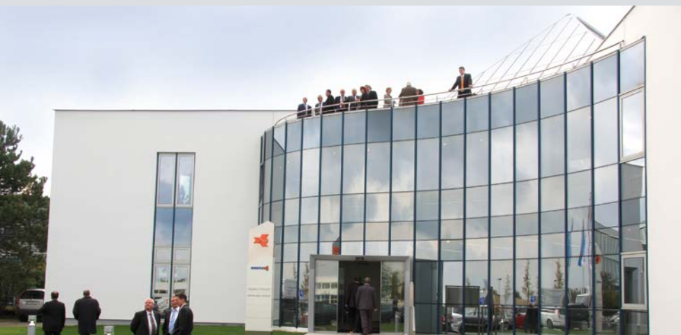
In 2008, SWARCO inaugurates a new corporate building in Perchtoldsdorf near Vienna, workplace for roughly 80 employees.
