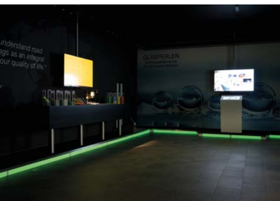
Escape route markings with afterglow
