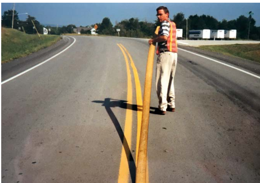
Jon Sproul, today SWARCO's General Manager for the US road marking materials operations, removing temporary tape for roadwork zones
