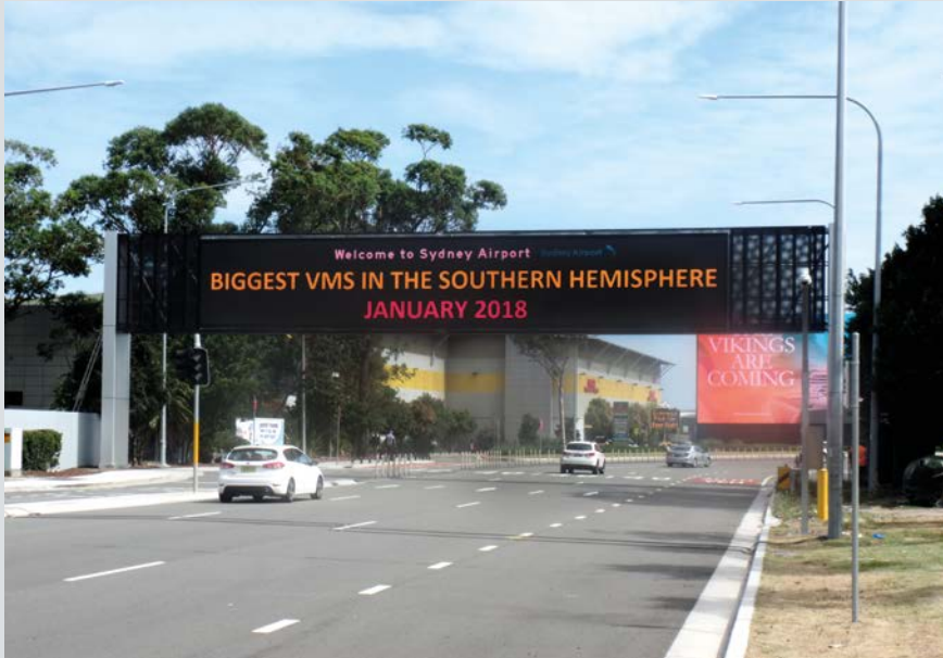
Giant information panels made in Austria for Sydney Airport in Australia. 750,000 LEDs consume less energy than a standard vacuum cleaner.
